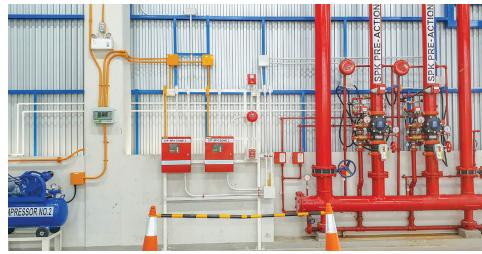
This type of system uses pressurized air in the pipe—or sometimes nitrogen—which provides the necessary pressure in the pipe to keep the check valve closed.
